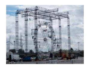
The wheel was constructed in sections which were floated up the river Thames on barges and assembled lying flat on pontoons. Once the wheel was complete it was raised into its upright position by cranes, initially being lifted at a rate of about 2 degrees per hour until it reached 65 degrees.
